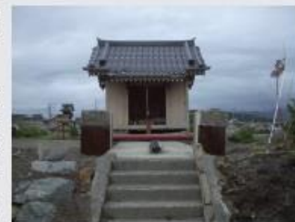
A small shrine in Hisanohama. The area around it was completely destroyed but the shrine remained. The large red torii gate leading to the shrine had collapsed.
