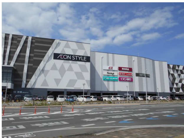
Aeon Mall Iwaki-Onahama, a shopping centre designed to double as a short-term shelter facility in case of disaster
