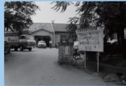
Left: While the new city hall building was being built, the former Taira Commercial High School site was used as a temporary Iwaki City Government building. (Photo by Iwaki City 1969)
